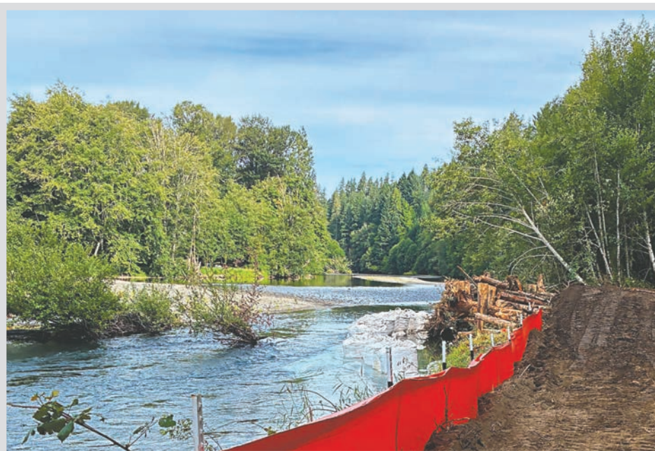
Deflector jam with cofferdam
