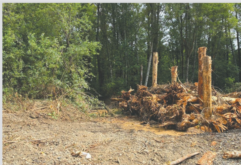
Log jam at side channel outlet
